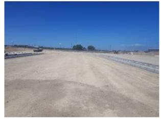
Image 32: Compacted area, awaiting paving.
