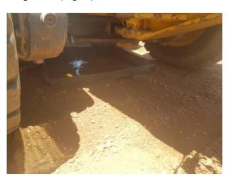
Image 16: Drip tray placed under stationary construction vehicle. Image 17: Stockpiled material on site.
