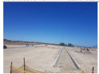
Image 13: Laying of pavement curbs on site.
